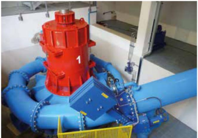
Peltonturbine 5-düsig, 450 kW, Val di Sole (Italien-Trient)
